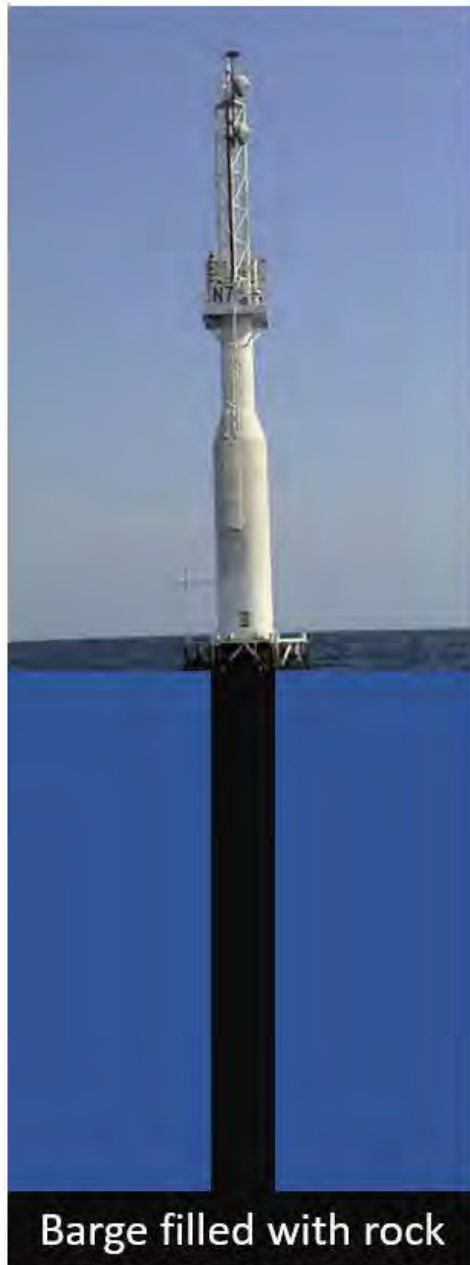
Figure 2. Basic Structure of the Northern Gulf of Mexico Air Combat Maneuvering Instrumentation Towers
